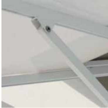
Scharniere einzeln verschraubt. Hinges are bolted separately.
